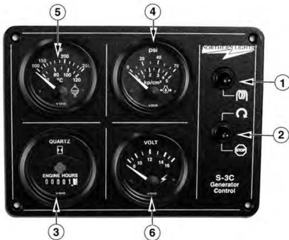
Figure 3-B: Series 3 Generator Control Panel
